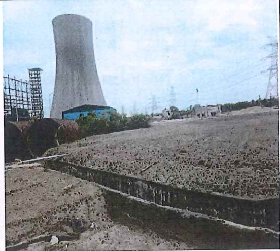
b) Bottom ash from the clinker utilized for filling low lying area with the unit's premises
